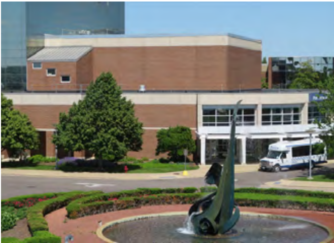
Achieving OSHA roofing safety requirements does not mean that your building needs to look like a construction site. This community college facility meets OSHA guidelines, yet the fall prevention and restraint systems blend in.
