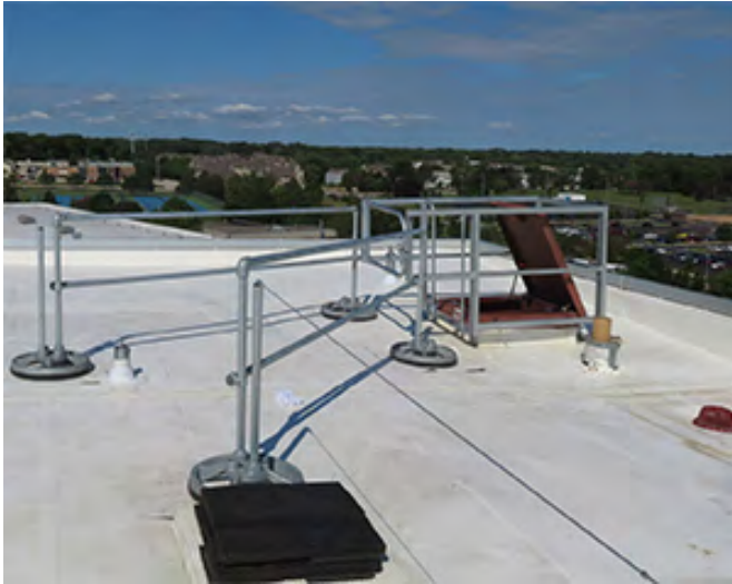
Roof hatches require rails on three sides—the hatch cover protects the fourth side. This allows the employee to put one hand on a side rail while using the other to open the gate.
